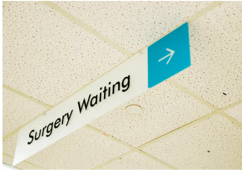
Absorptive ceiling tiles reduce the volume of sounds reflected off their surfaces, the length of time they last, and distance they travel.
